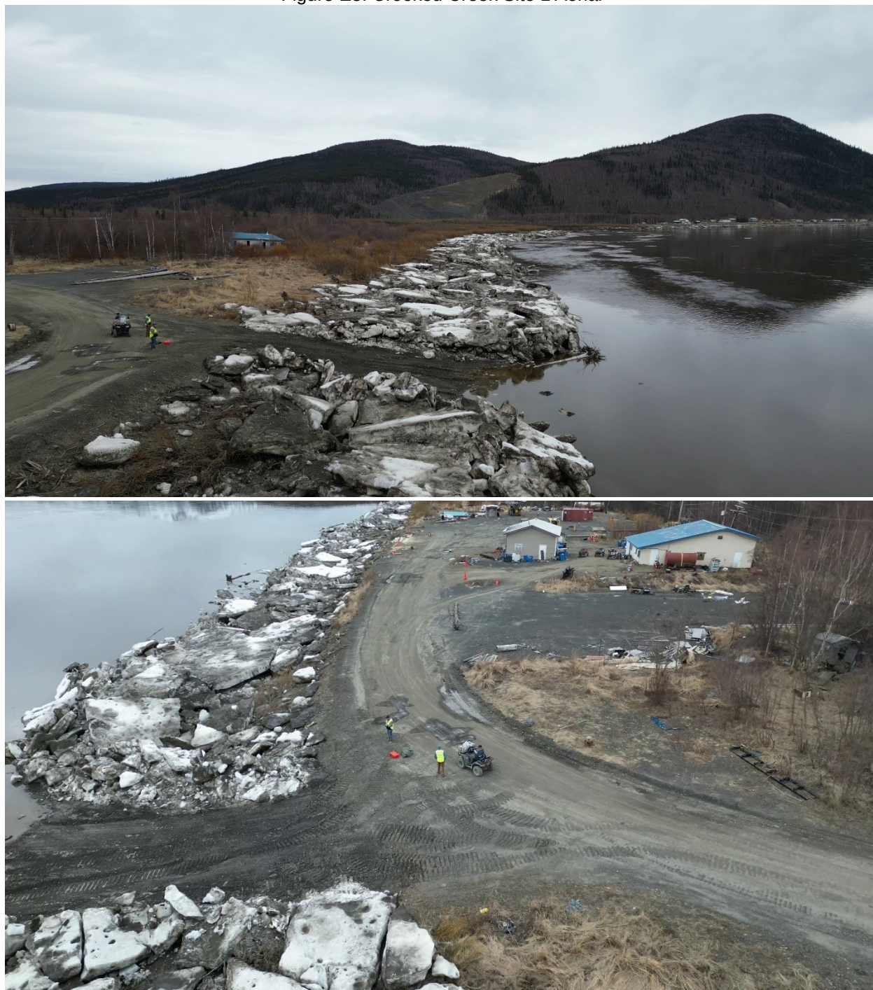
Figure E3. Crooked Creek Site 1 Aerial
