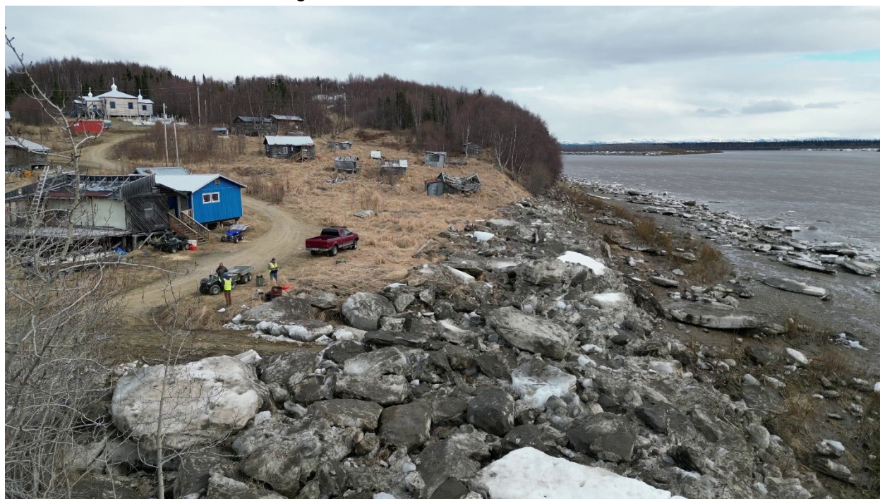
Figure D4. Chuathbaluk Site 1 Aerial
